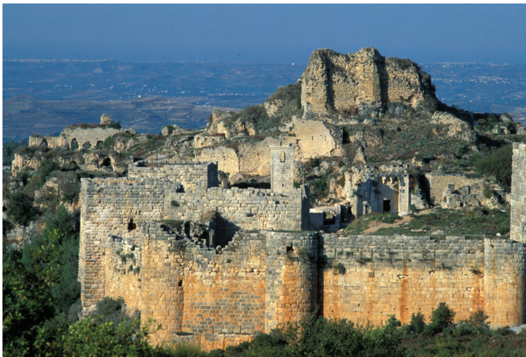
Plate 36. Sigon (Salah ad-Din). View of the fortification.
